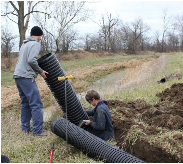
Installation of a water control structure.
