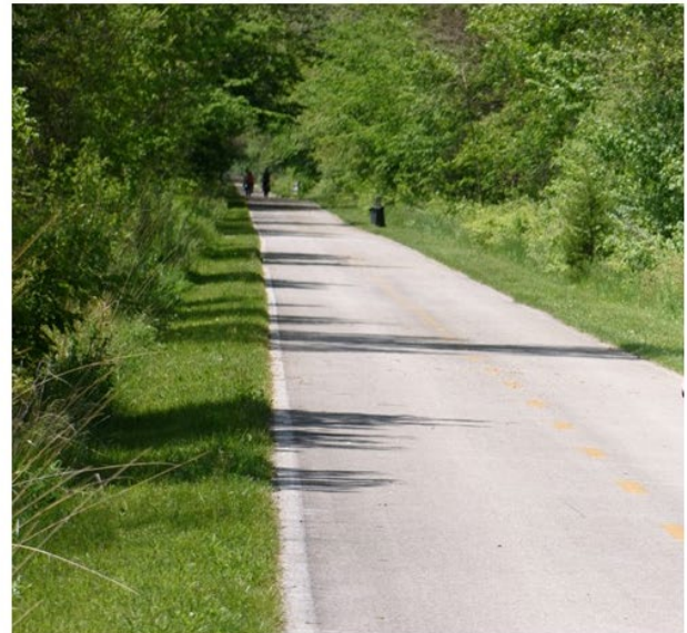
A surface view from the trail; Source: Photo courtesy of Metroparks Toledo, May 2020
