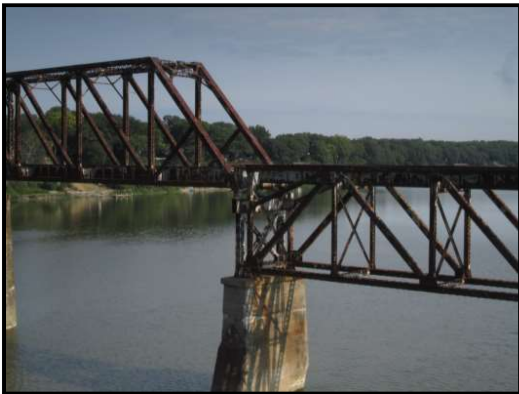
Figure 3: Transition from Deck Truss to Through Truss
