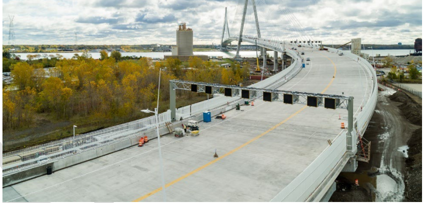
Source: Windsor-Detroit Bridge Authority, 2025; https://gordiehoweinternationalbridge.com/gallery/photo-gallery/bridge-site-progress-november-2025/
