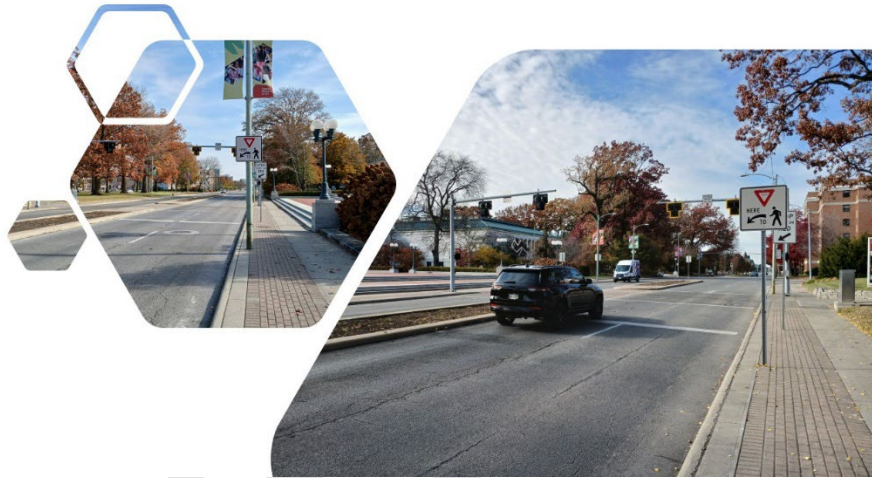
Pedestrian Yield Signs associated with a HAWK beacon, outside the Toledo Museum of Art, Monroe Street, Toledo, Ohio
