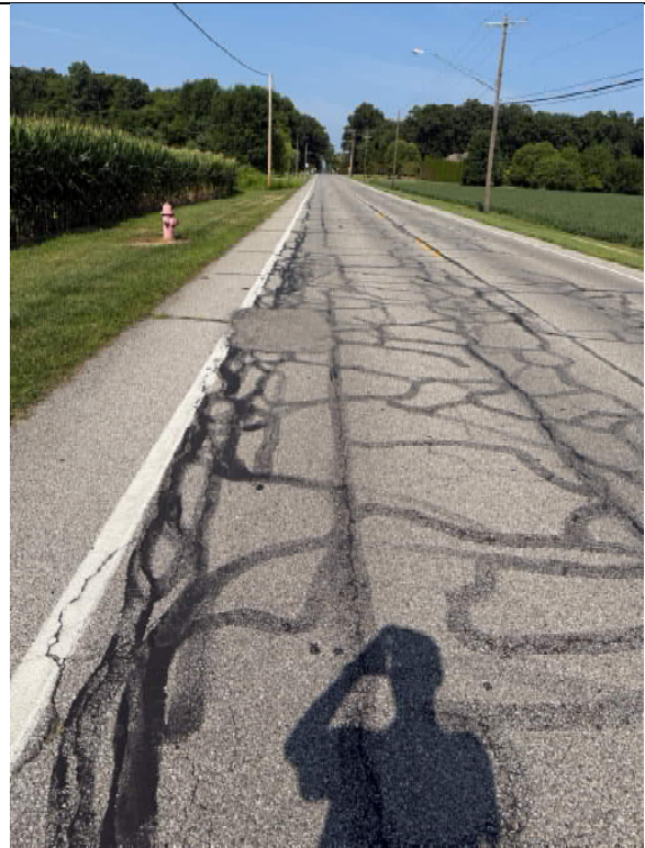
Photo 2 Waterville St., looking west
