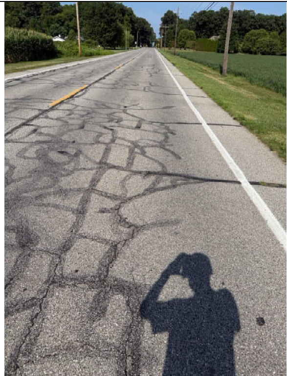
Photo 4 Waterville St., looking west
