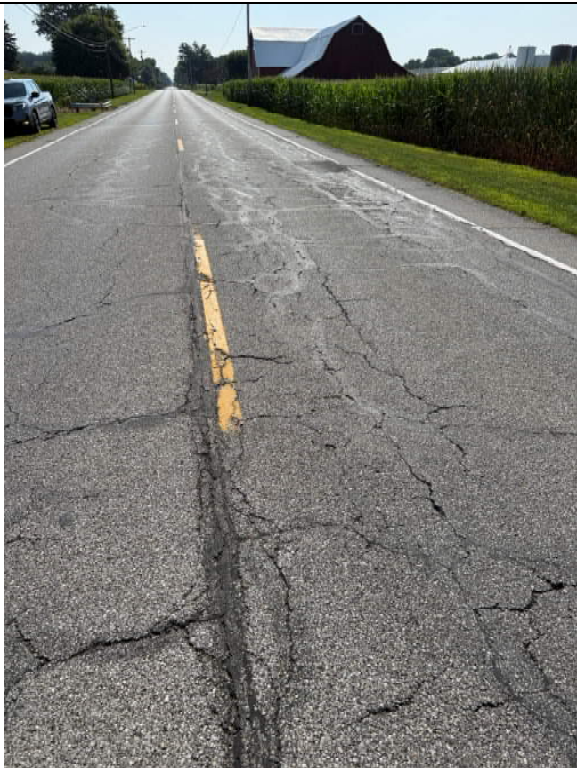
Photo 3 Waterville St., looking east
