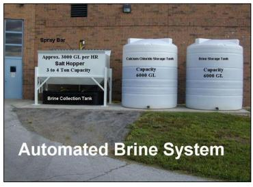
effective working temperature in colder conditions. Additionally, these same liquid chemicals can be applied directly to the pavement in both anti-icing and de-icing applications.
